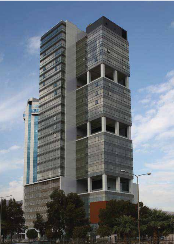
● MEGAPOL TOWER / IZMIR, TURKEY
